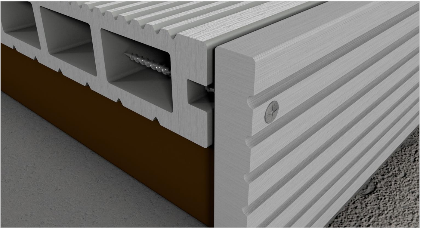
Figure 18: Installation of the Skirting Board with Self-Drilling Screws
